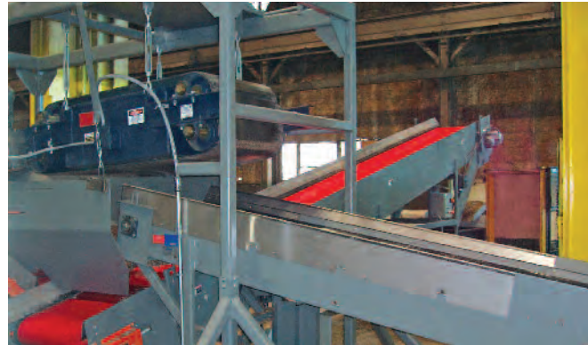
Magnetic Metal Separation System
