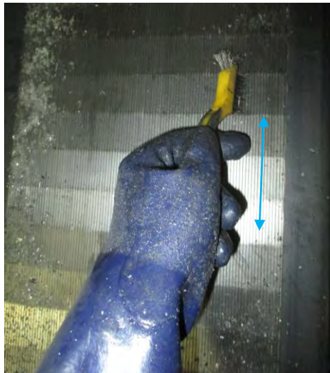
Figure 22: Scrape Filter
