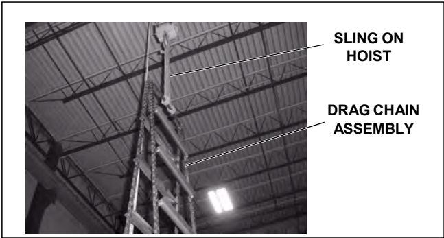
Figure 9. Lifting Drag Chain Assembly With Hoist
