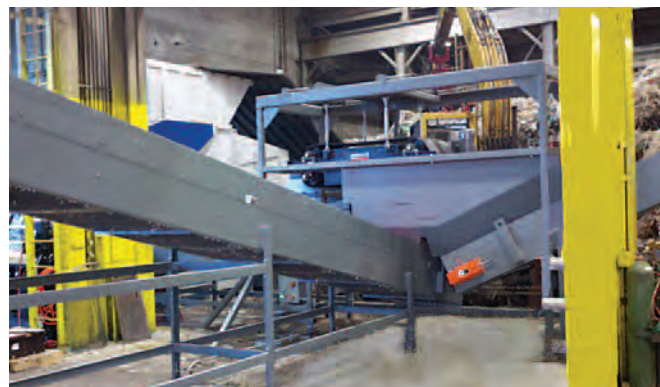
Slider Bed Transfer Conveyor working at a plastics recycler
