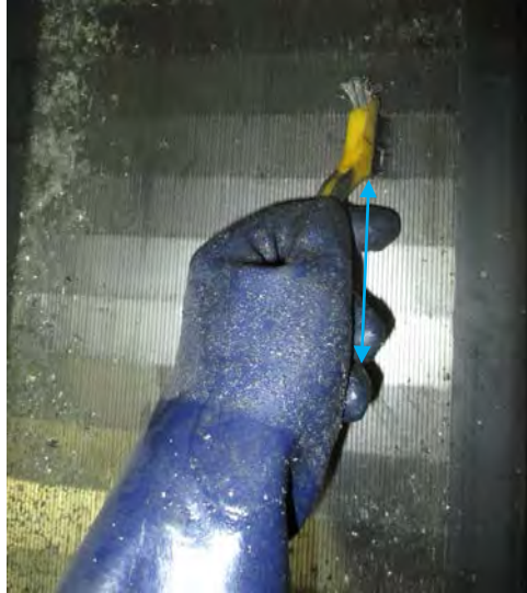
Figure 22: Scrape Filter
